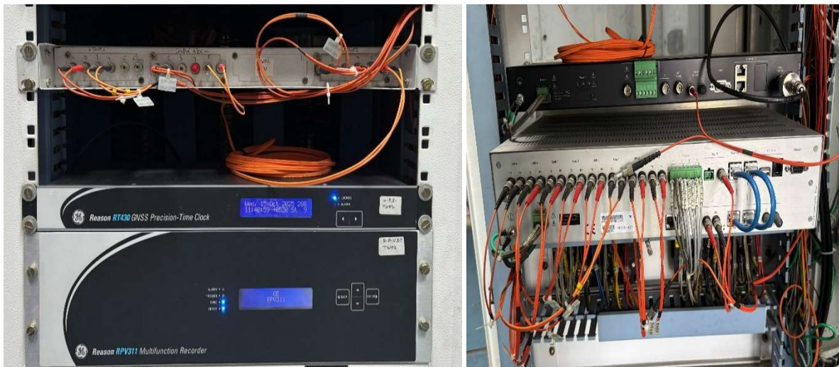
Figure 2: Decentralized Architecture of GE make TWFL
